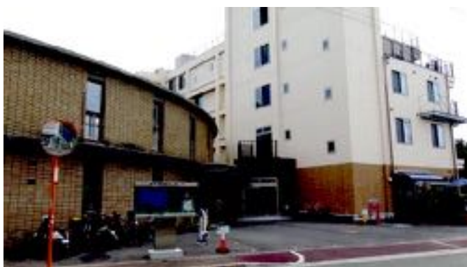
Left – Church building Right – Aged Care facility
